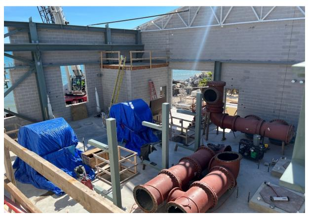
In the coming months the pumpstation will be outfitted with four vertical turbine pumps with a total pumping capacity of 36MGD, HVAC system, dual backup generators, chemical feed system, security system, and Supervisory Control and Data Acquisition (SCADA).
